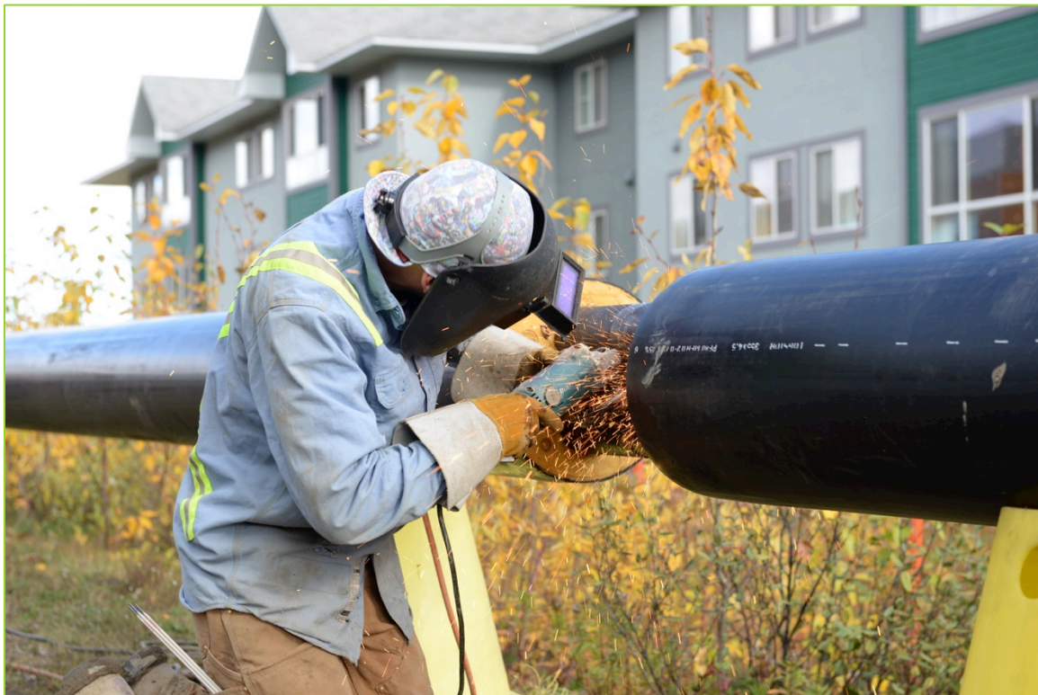
Figure 1 - A worker prepares the pipe for the Sustainable Communities Demonstration Project
